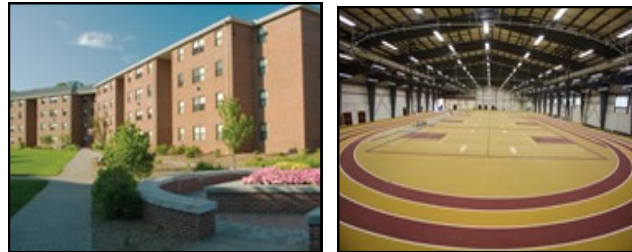
Residence Hall and Field House
